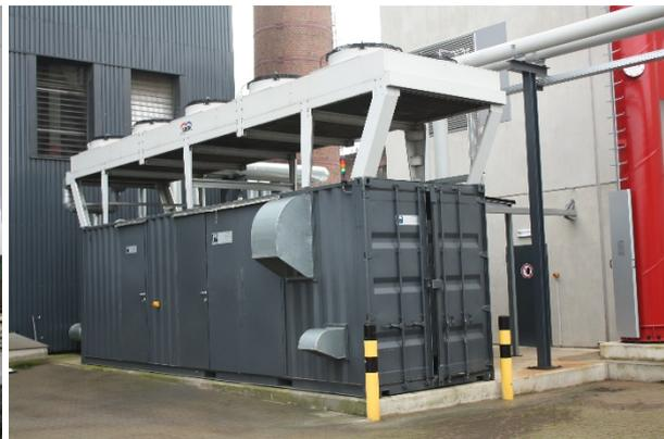
Left: Cabero adiabatic dry coolers for cooling of the E-RATIONAL ORC – Right: E-RATIONAL ORC machine in container
