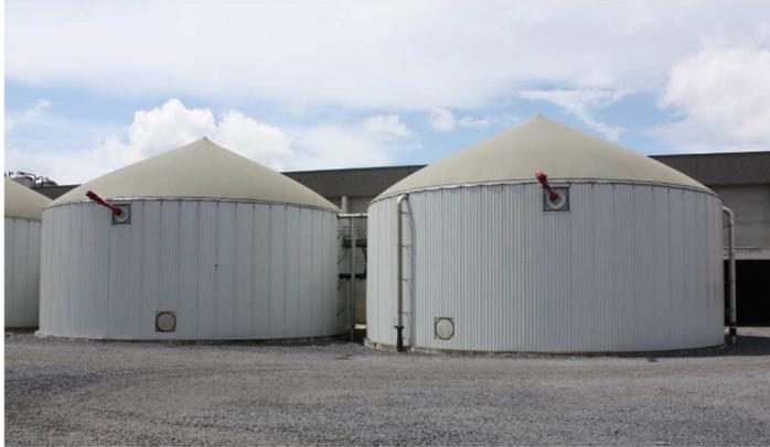
The green power from the plant is fed into the grid. The heat from the motor jacket cooling and the exhaust air is used to heat multiple parts of the plant, such as the digesters themselves, the offices, the pasteurization process, drying of specific waste streams and other facilities on the site. The digestate of the fermentation process is applied as a soil supplement in agriculture and horticulture.
