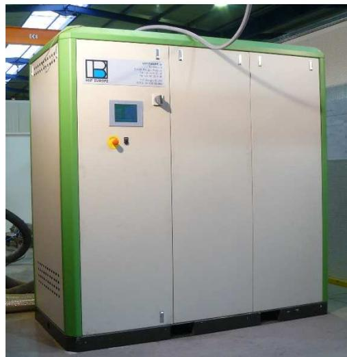
Instead of using electricity to dump the heat excess through coolers, the ORC is producing electricity available for consumption on the site.
