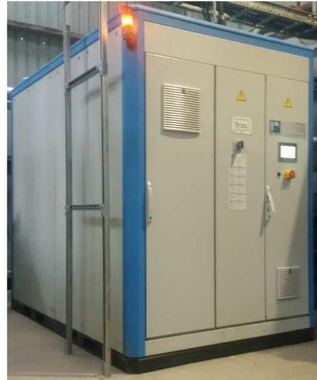
Hot water at 130°C is produced by the biomass boilers and sent to the ORC machines. The return temperature to the boilers is 115°C. The cooling water circuit of the machine operates at 35°C inlet to 45°C outlet temperature and warms the air blown by the fans on the drying floors. Average net power production of each E-RATIONAL ORC machine at full load is around 75kWe.
